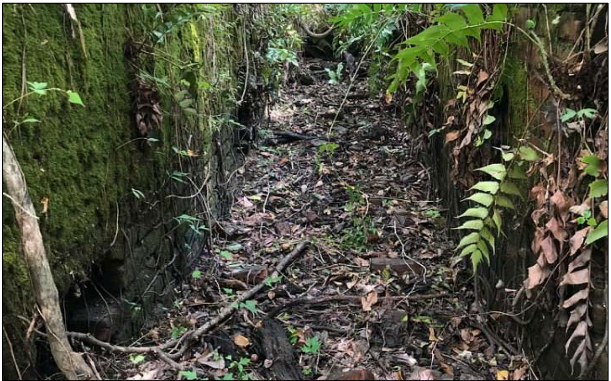
Figure 5.38. View of area between features A and B, facing northeast.
